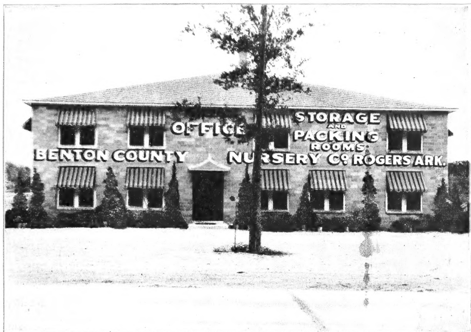
Our New Office and Storage House—The Most Modern in the Southwest
